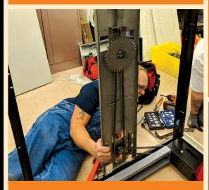
Technicians from Tyler Supply Co. retrofitting the storage unit to manual assist operated by a chaindrive system.
